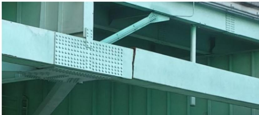
May 11, 2021 a fracture was discovered in one of the main span tension ties at the location of a butt weld in the I-40 Hernando de Soto Bridge, Arkansas/Tennessee.
